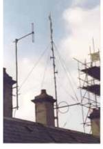
off in RX performance. Dire thoughts about RX antenna problems and other expensive faults were raised when Mark 'SDR went on site to test RX sensitivity and found this OK. Even more head scratching when it was reported that the RX ant was showing a VSWR of over 3:1!
