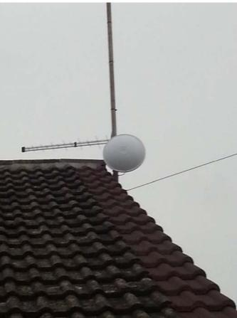
Completed installation of the small 5GHz Dish at the Lansdown Repeater site.
