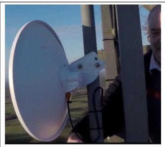
Connection to the new dish was made while Mat carried out some checks on the ground to make sure that he could communicate with the new 5GHz transceiver and to confirm the correct channel, Rx noise floor level and Tx power of the link. During this time adjustments to the dish's alignment were made to insure we were firing at the right bearing and down tilt.
