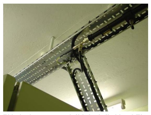
This is a shorted quarter wave co-ax stub with the shorted end bonded to earth. This should help keep noise, rain / storm static and any lightening discharges from building up on the feeder and possibly discharging into the Tx/Rx units.
