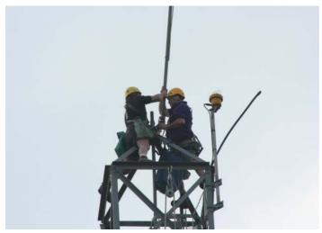
Old antenna being removed from the top of the tower.
