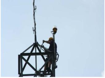
New antenna fitted, just waterproofing the connector.
