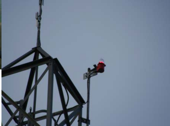
Left: New LED type lamp fitted January 2013.
