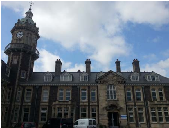
The frontage of Cossham Hospital after revamp.
