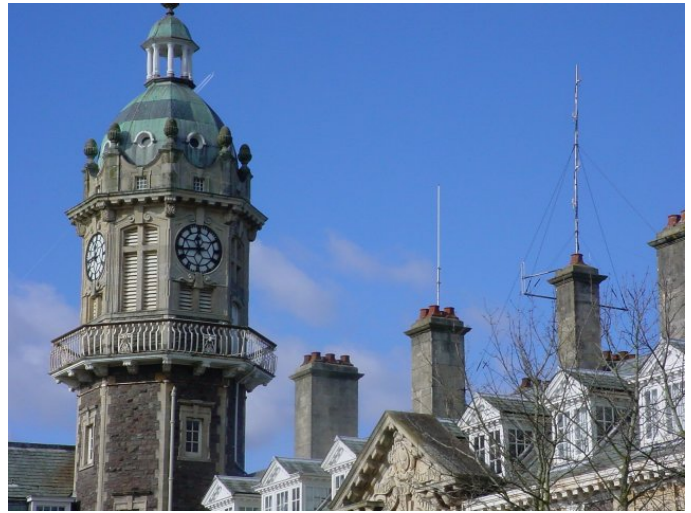
Cossham roof line, including the old GB3BS Antenna.
