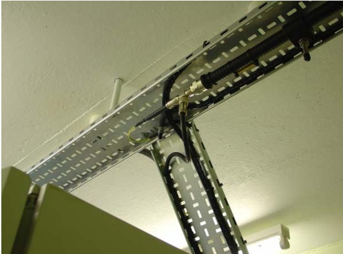
This is a shorted quarter wave co-ax stub with the shorted end bonded to earth. This should help keep noise, rain / storm static and any lightning discharges from building up on the feeder and possibly discharging into the Tx/Rx units.
