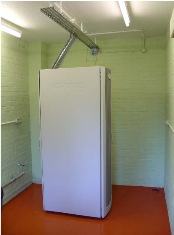
The shiny new floor, cabinet and tray work
