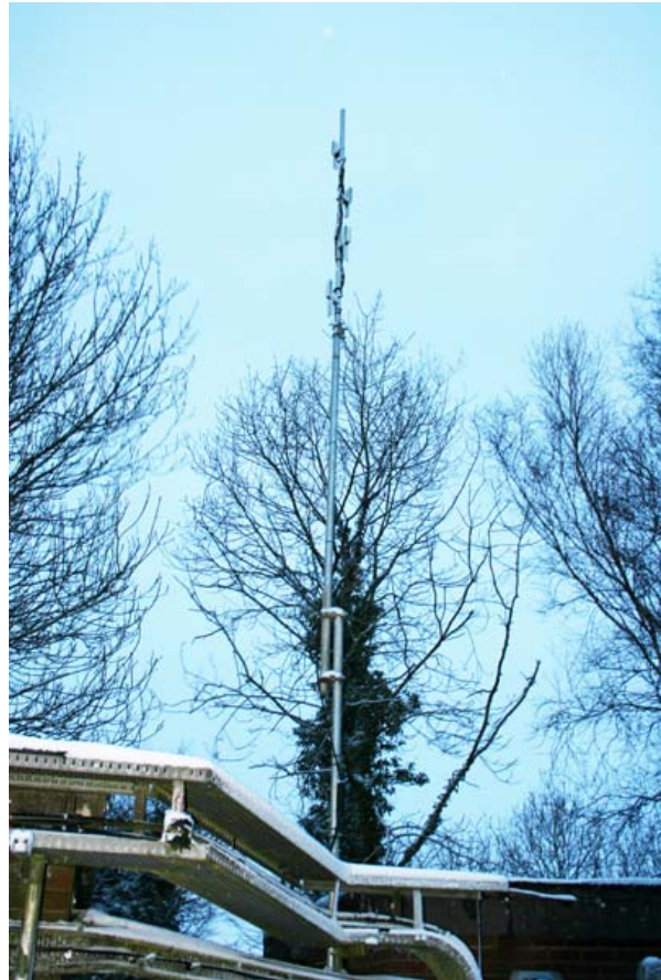
Temporary antenna system at its full height
