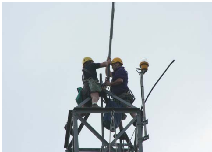
Old antenna being removed from the top of the tower.
