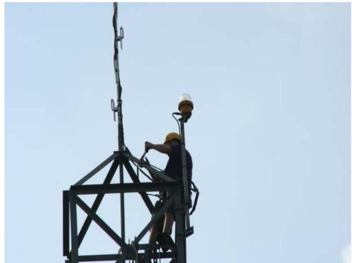
New antenna fitted, just waterproofing the connector.
